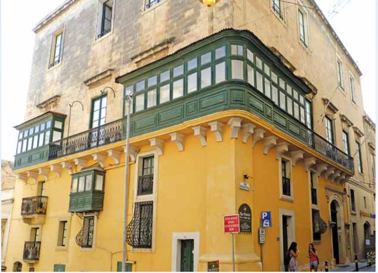
A knights townhouse in Valletta with its characteristic traditional painted walls and wooden painted balconies.
